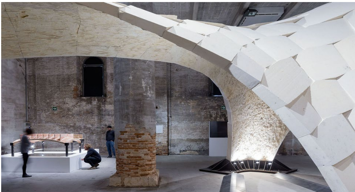
Fig.04. The Armadillo Vault – A grand piece of modern application of stereotomic principles using CAD and CAM by the Block Research Group.
